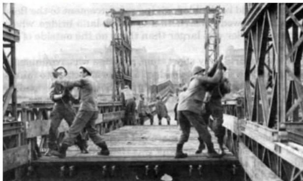
Class 70 Bascule Bailey Bridge being raised
