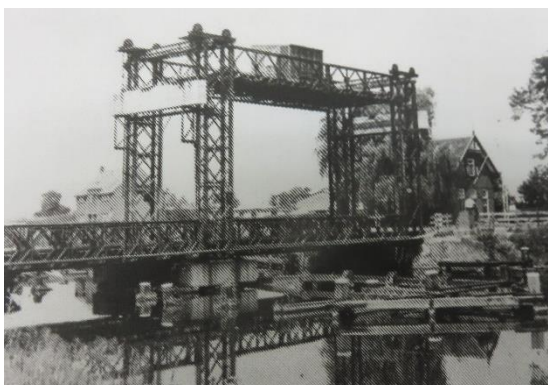
Class 70 Bascule Bailey Bridge being raised
